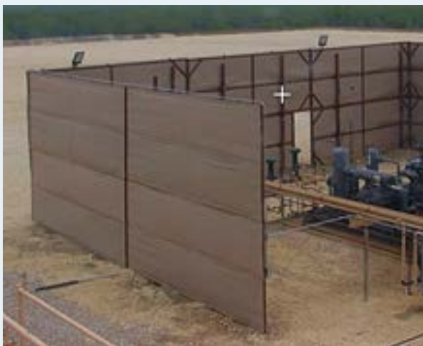
Sound barrier installation at Eagle Ford Shale
